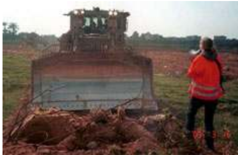
Picture taken between 3:00-4:00PM on 16 March 2003, Rafah, Occupied Gaza. A clearly marked Rachel Corrie, holding a megaphone, confronts the driver of one of two Israeli bulldozers in the area that were attempting to demolish a Palestinian homes. She was confronting the bulldozer in order to disrupt its work, and prevent it from threatening any homes. Photo by Joseph Smith. (ISM Handout)
